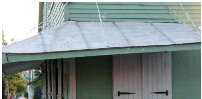
This canopy includes a standing seam metal roof. Canopy supports should be reviewed periodically, particularly where canopies are not level, to ensure they are well supported and not in danger of collapse.
