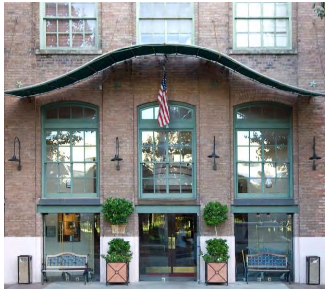
An example of a major character altering alteration is the new entrance added at the ground level of this building while maintaining the historic window openings above. Minor alterations include the new canopy and lighting.
