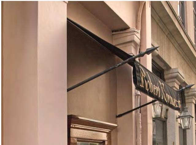
The awning is mounted between the granite piers. The poles are fastened to the stucco surface rather than the masonry, facilitating future repair if removed.
