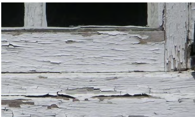
The window sill and jamb have peeling paint and some checking or splitting. Removal of the loose paint will allow the wood to be inspected for signs of rot.
