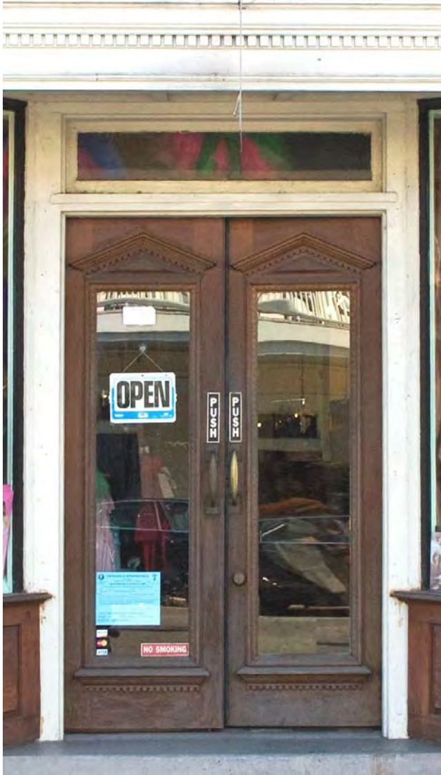
The paired door includes large glazed panels with a decorative pediment and is topped by a transom window.
