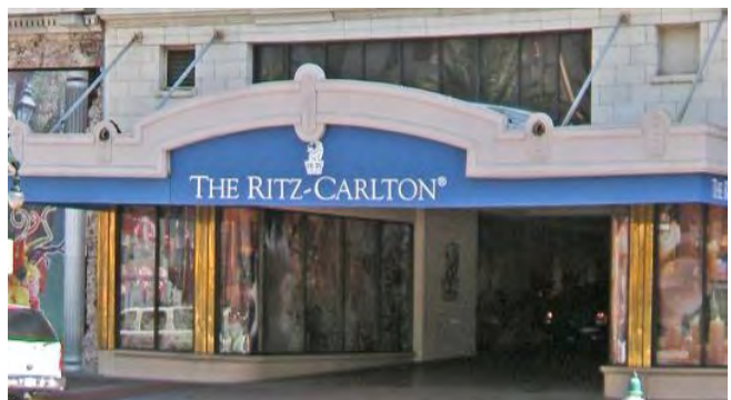
This canopy includes a standing seam metal roof. Canopy supports should be reviewed periodically, particularly where canopies are not level, to ensure they are well supported and not in danger of collapse.
