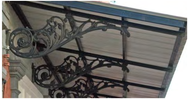
Decorative cast iron brackets and a frame support tongue and groove decking with standing seam roofing above.
