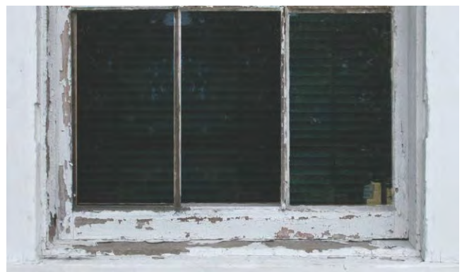
Typically, window deterioration first occurs at the sill. Peeling paint can allow moisture to enter wood and cause rot.
