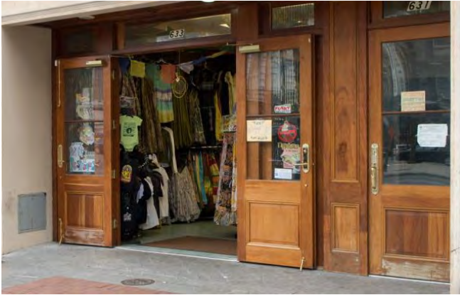
A new wood storefront was installed that includes transom windows, sidelights, glazed paired entry doors and a secondary door to access upper building levels.
