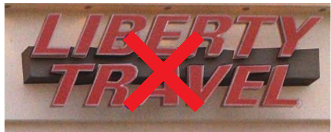
Exposed raceways for channel letter signage are not permitted.
