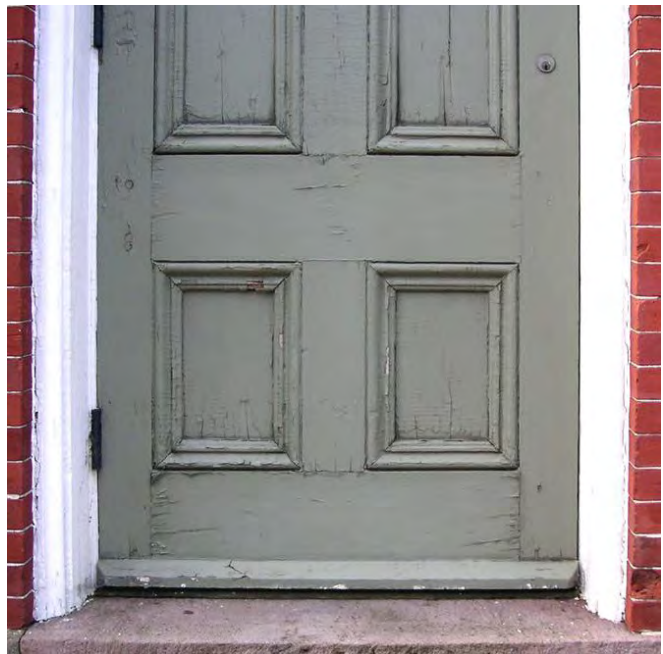
Wood checking (splitting) and peeling paint visible. Minor repair and maintenance can prolong the serviceable life of this historic door. The trim at the bottom rail of the door helps prevent storm water from entering the building.
