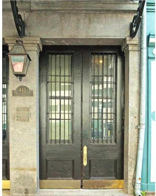
The granite lintel is structural, spanning between the flanking Greek Revival pilasters.
