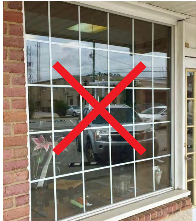
Example of an original storefront window opening that has been incorrectly filled with a vinyl, simulated divided-lite window.
