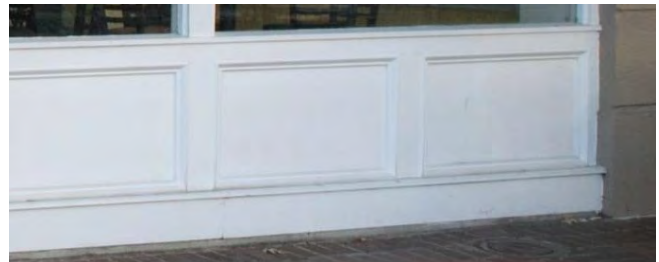
The vertical mullion divisions in the window above correspond to the wood panel divisions at the bulkhead below.
