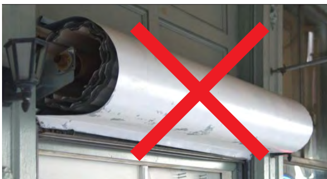
Exterior security grille housings are not permitted.
