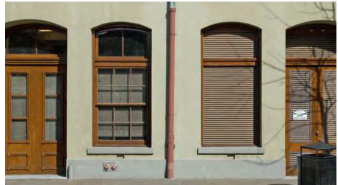
The rhythm of the storefront was maintained in the installation of the building equipment behind the louvered window and door.
