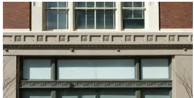
The storefront cornice visually separates the storefront from the upper building levels.
