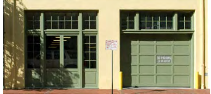
The former storefront opening to the right was modified for use as a garage. The historic transom window configuration matches the storefront to the left.
