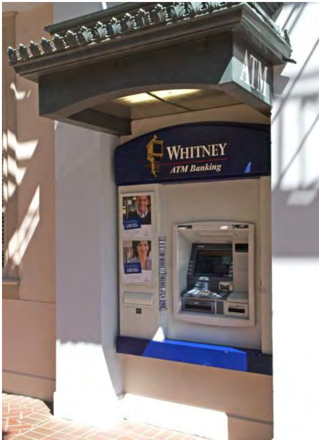
This ATM canopy was designed in a manner that complements the building's style and includes integrated down-lighting illuminating the immediate area allowing the merchandise to be visible when the store is closed.
