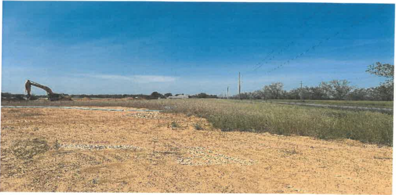
9. In the process of installing utilities on the north section
