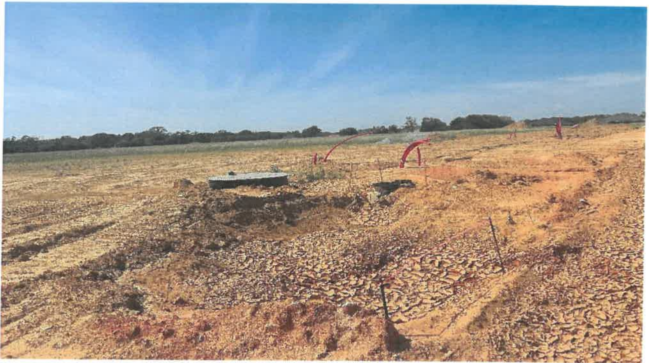
12. Stormwater infrastructure in place & manholes
