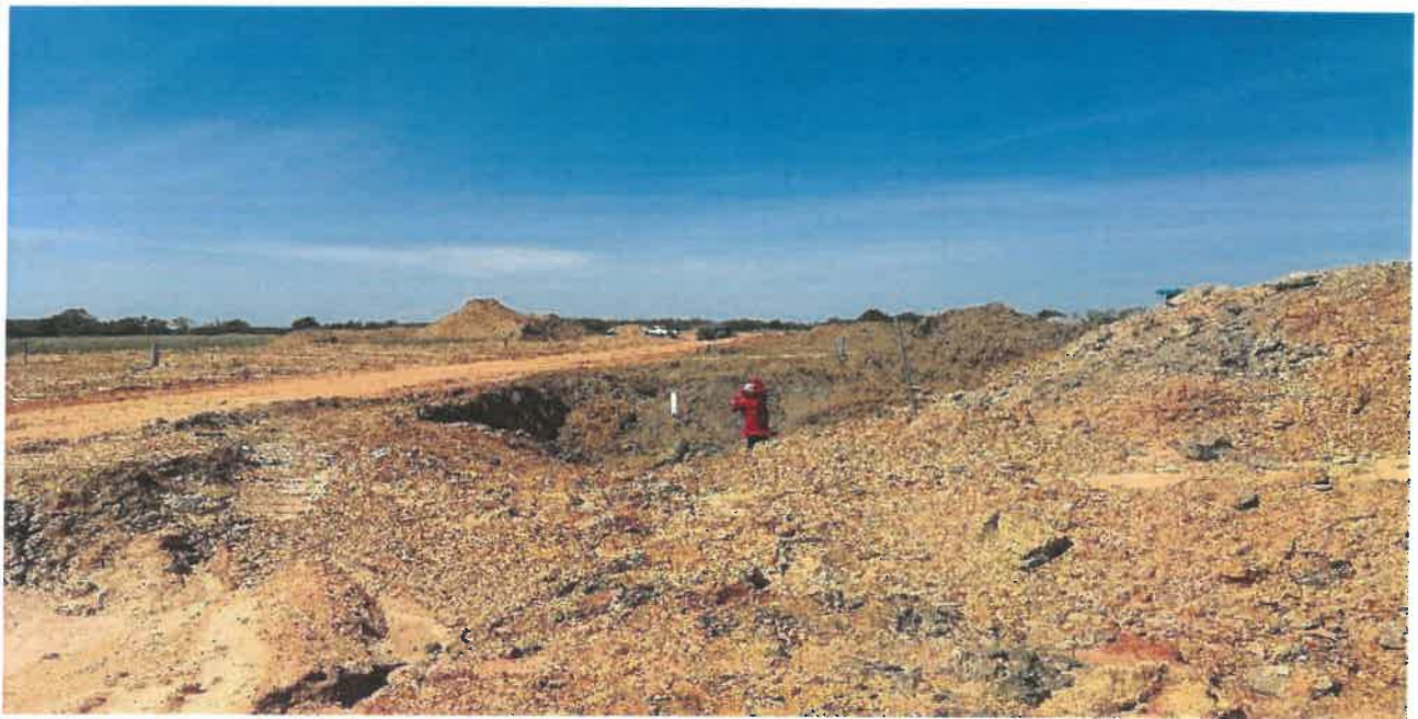
2. Hydrants in process of being installed
