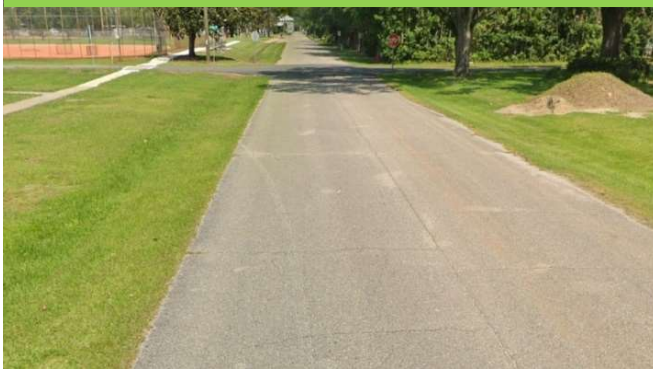
West Roosevelt Avenue from Cedar Street to SR-59
